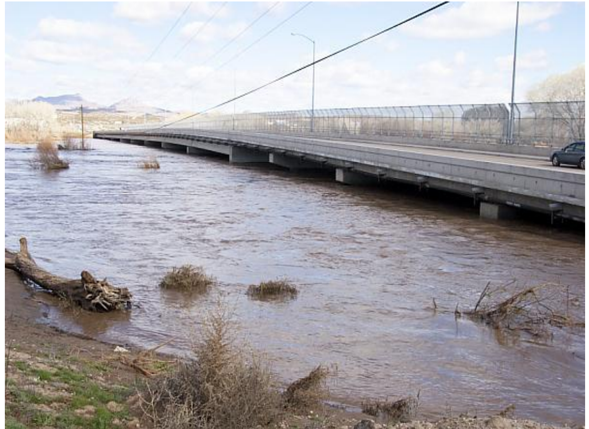
Figure 3: Bridge Crossing the Gila River in Duncan, AZ [5]
