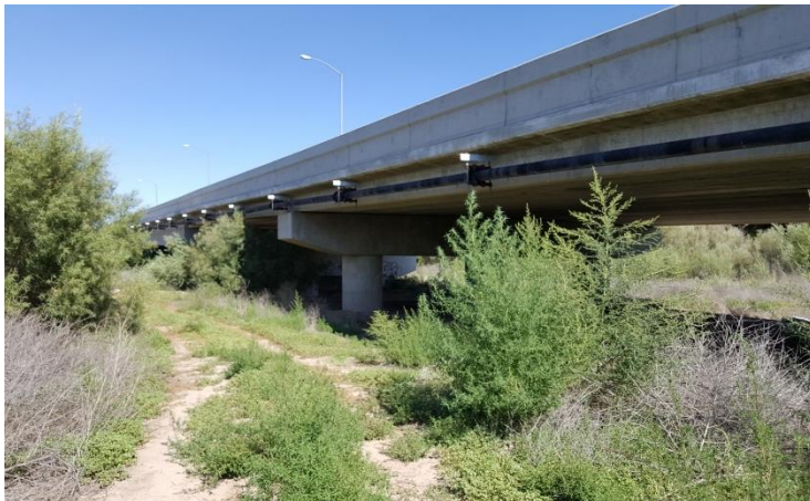
Figure 8: Downstream view of bridge
